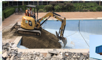
Construction crews filling in the pool to make space for the courtyard (above) and replacing the roof at Compass Point Village (right).
